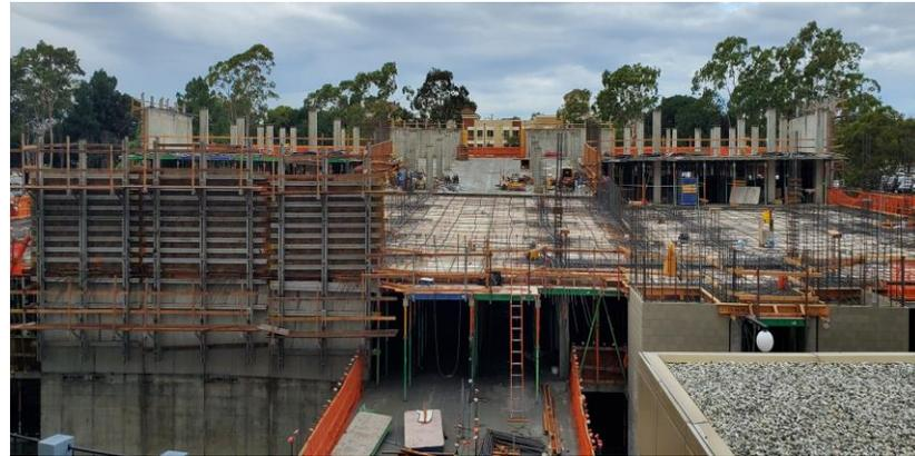
Construction continues with the parking structure. East deck concrete pour for level four is scheduled for 1/3/20 with columns and wall concrete pours following on 1/14/20.
